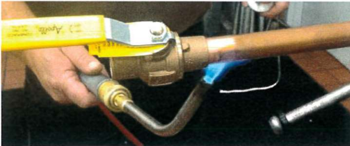
Figure 1 - Preheat tubing
