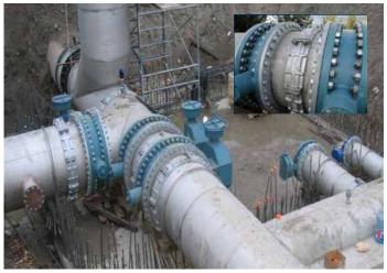
R-88 couplings used on a stainless steel hydro electric piping system.
