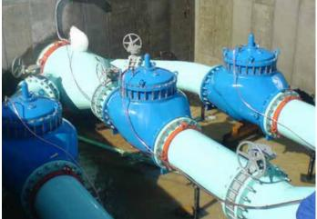
VSH Shurjoint Ring Joint couplings used in a water treatment application
