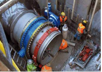
VSH Shurjoint Ring Joint R-88 couplings used in a domestic water treatment plant.
