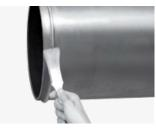
After welding apply a thin smooth coat of a rust prevention resin paint coating to the rings, weld areas and pipe ends. A fast drying paint is preferred.
